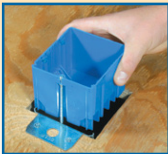
Install clip over subfloor.
