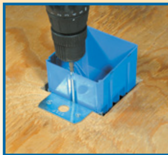
Screw in to adjust to height of flooring or carpet.
